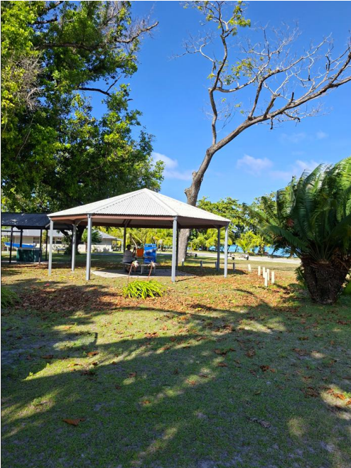
Figure 2: Replaced roof and battens at Tourism shelter at Home Island
