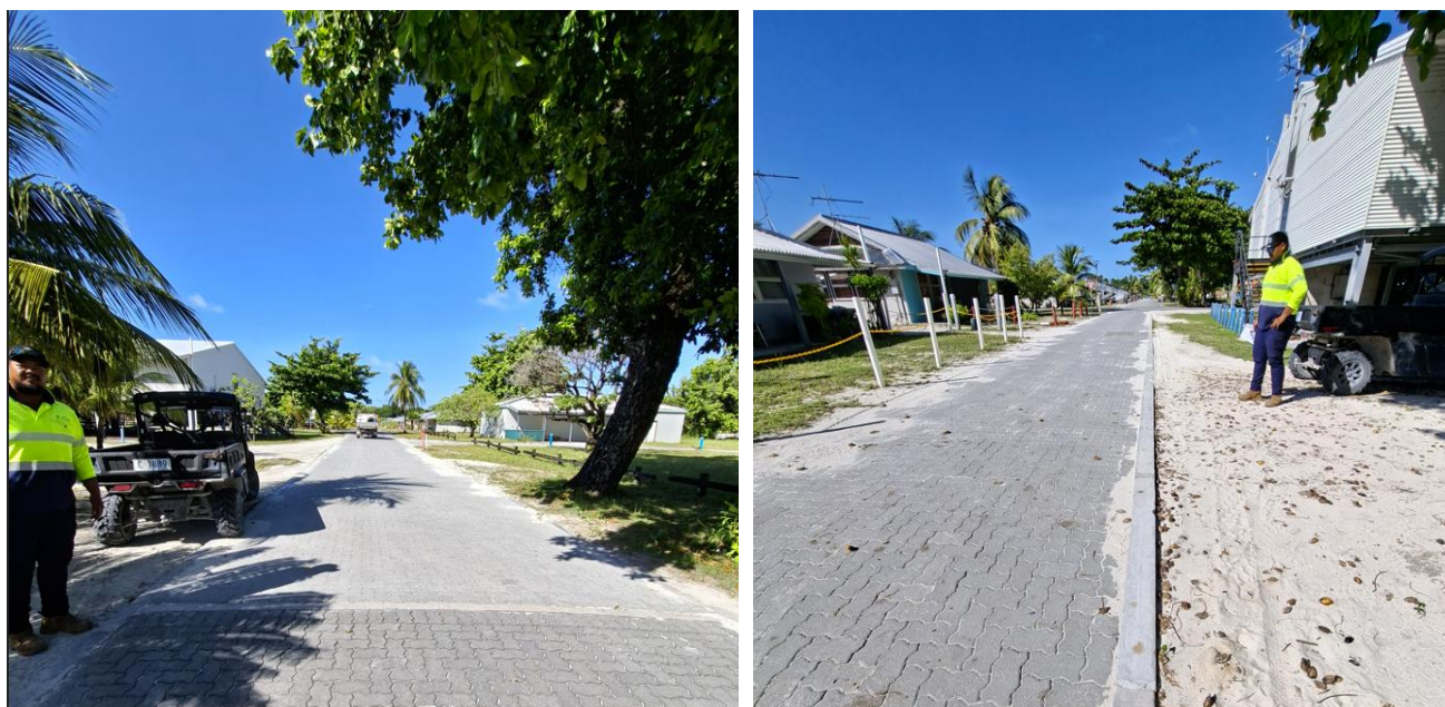
Figure 4: Sections of road paving was replaced and broken concrete edge strips were repaired on streets on Home Island.
