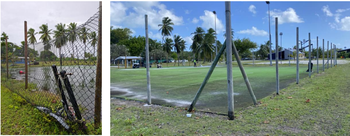
Figure 1: Removal of tennis court fencing and cleaning of surface.
