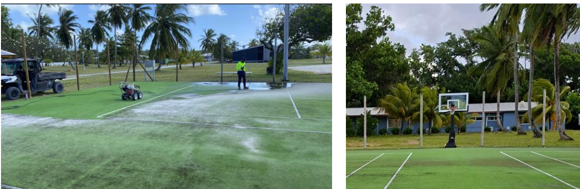
Figure 2: Cleaning of tennis court surface. Including a full size basket ball court and hockey/mini soccer pitch is being investigated.
