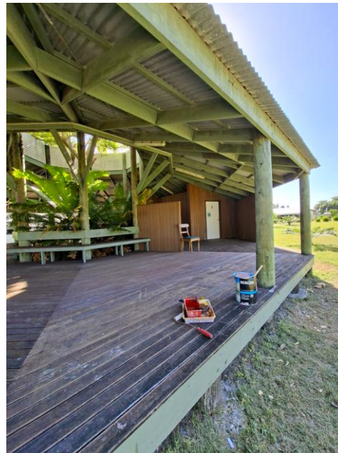
Figure 3: Commenced repairs on community Pondok next to Shire Office. Repairs included replacing wall cladding and varnishing of floors. Painting and replacement of the roof is still to be done.
