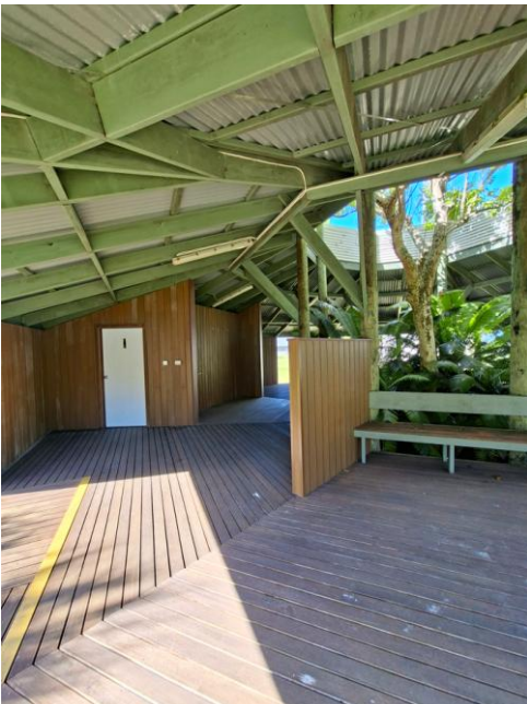
Figure 3: Commenced repairs on community Pondok next to Shire Office. Repairs included replacing wall cladding and varnishing of floors. Painting and replacement of the roof is still to be done.
