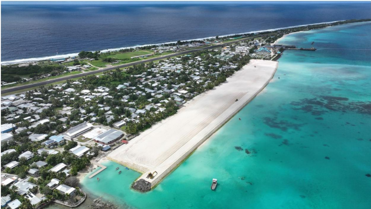
Figure 10-1: Coastal Hazard Adaption Works on Tuvalu
