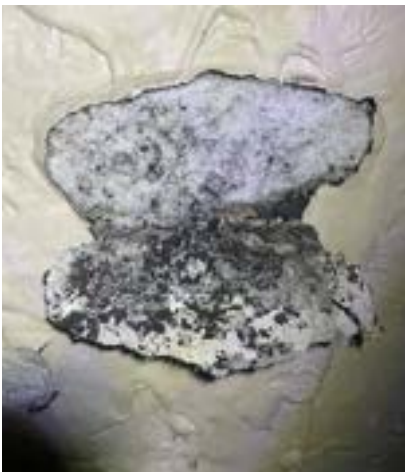
Salt Deposit underneath paint
