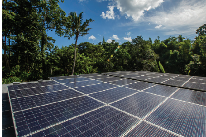
Solar panel power
